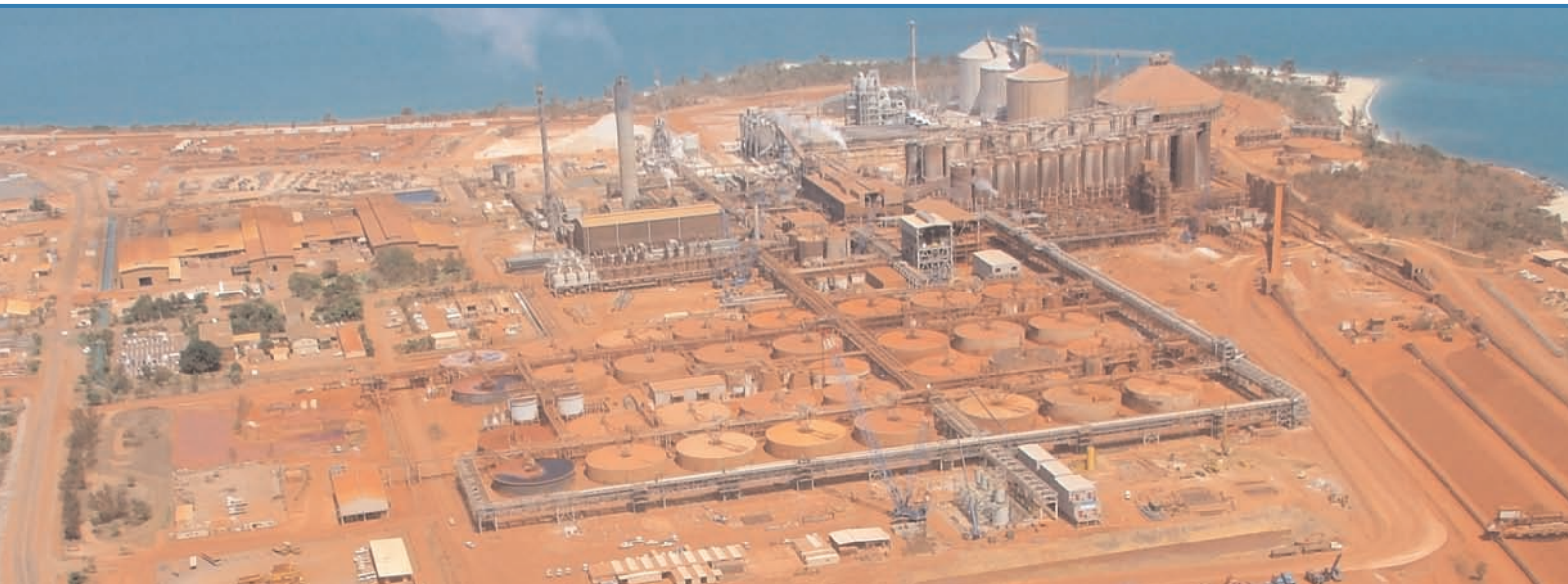
The Alcan Gove refinery at Nhulunbuy on the Gove Peninsula
