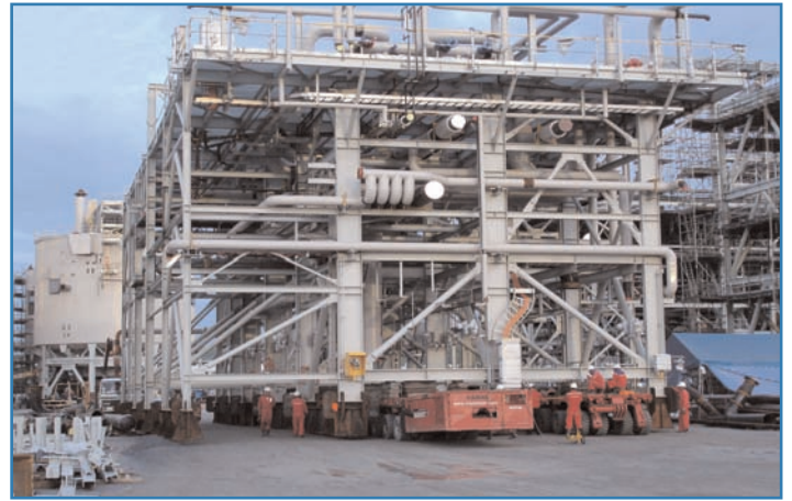
Loading operation of a PAM
